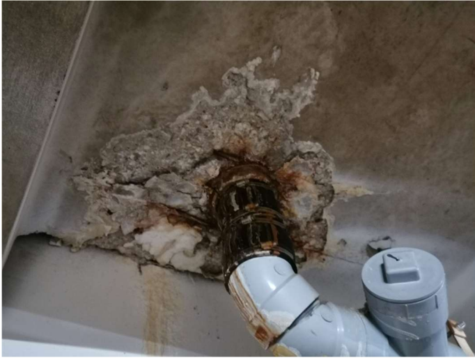
Parkade: Views of Previous Damaged Areas
