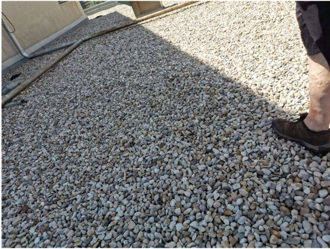
Views of Roof Surface
