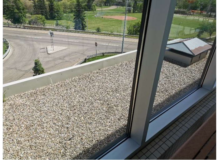
View of Roof Adjacent to Pool Facility (Main Floor)
