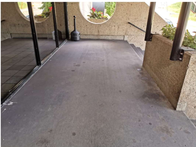
Main Entrance Exterior Landing
