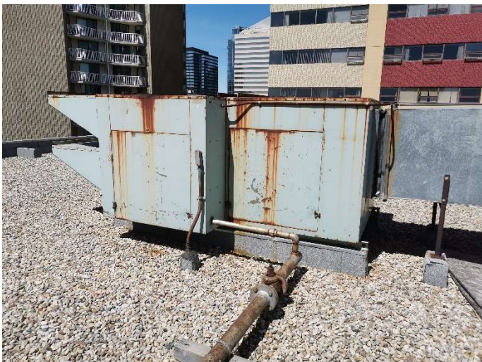
Makeup Air Unit, Example (Smoke Removal)
