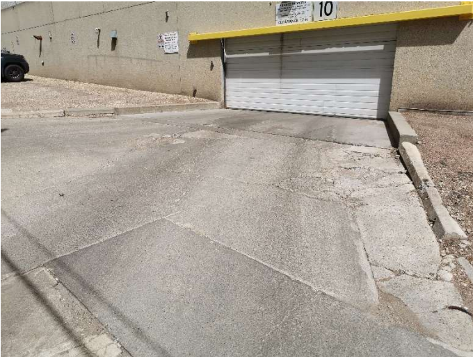
View of North Parkade Ramp
